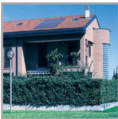
Example of sloped roof installation
