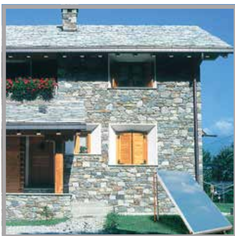
Example of ground installation
